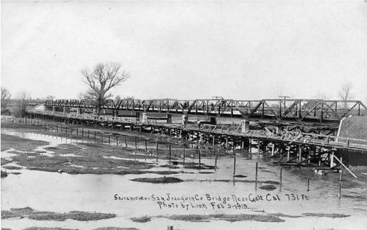
Photo dated February 5, 1910 showing temporary bridge used during construction of steel truss bridge seen in background.
