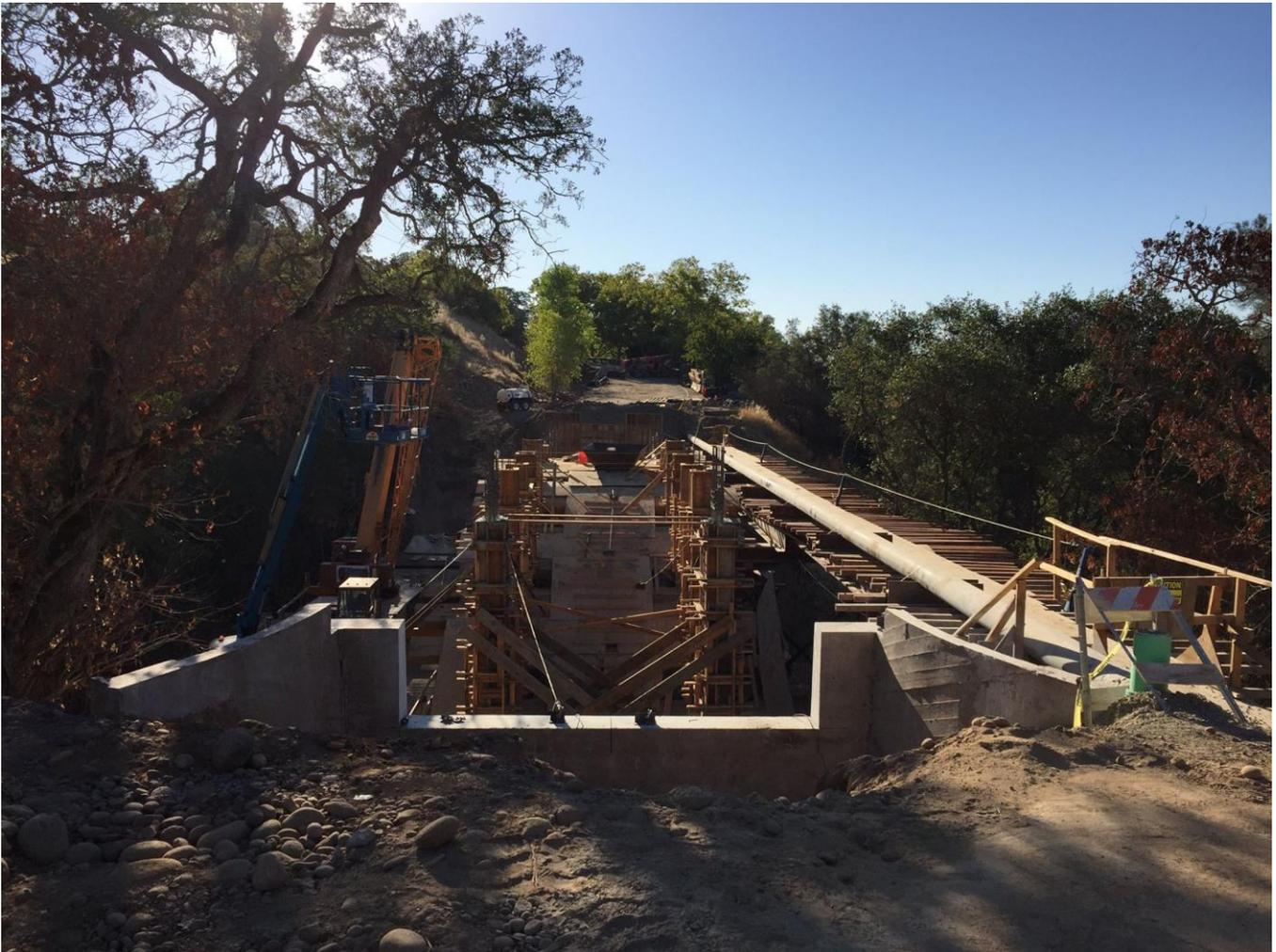
Photos taken by Joel Windmiller showing progress on deck replacement of Orangevale bridge
