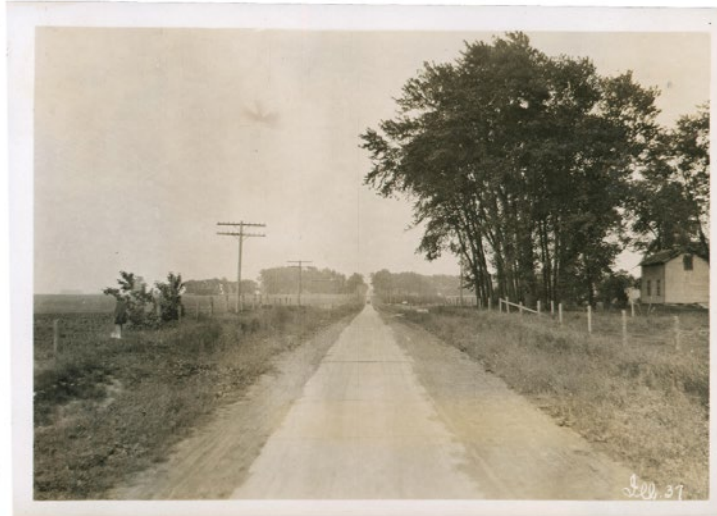
The first Seedling mile in the country at Malta, Illinois. The concrete pavement is 10 feet wide.
