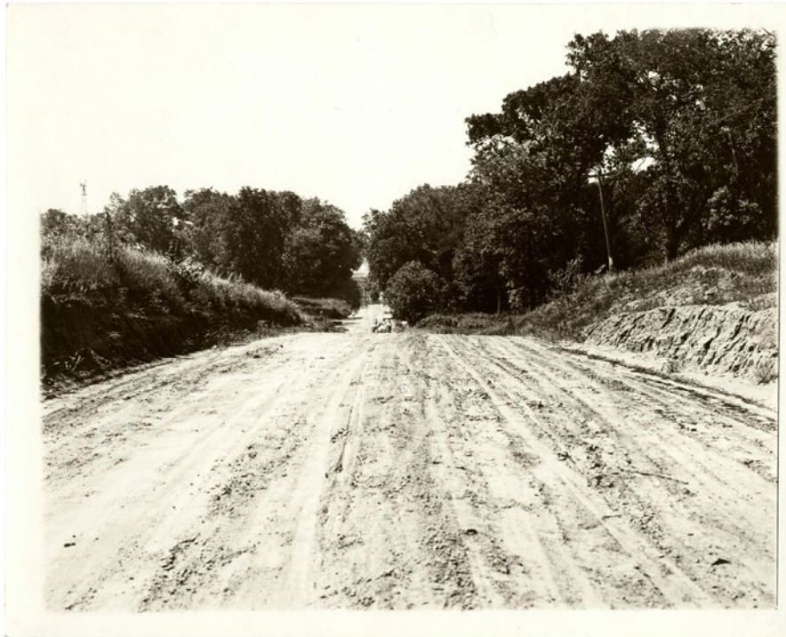
Looking west, seedling mile, Linn County, Iowa. Notice the depression in the road, which will be filled and the hill graded down
